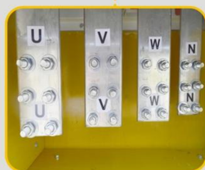
BUS BARS FOR LOAD POWER INPUT
